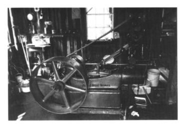
2. Cider Press - Boomer & Boschert No. 2; four 2 1/2" X 3 threads per inch power screws capable of being driven at three different speeds; 4'10" square racks with 96" square press cloths; maximum stroke of 48". Maximum capacity is approximately 10,000 pounds per day (1100 gallons). Manufactured in the mid 1890's.
